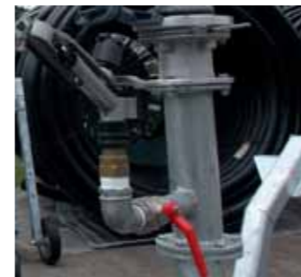
Second sprinkler on the trolley
