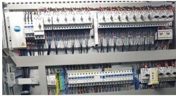
Picture No.14. Motor protection switches (top row) and fuses
