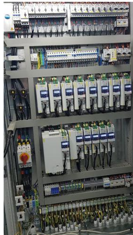
Picture No.4. Front inside view of Main – Motor control section cabinet
