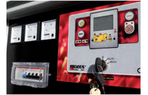
Control panel with ammeter, voltmeter and frequency
