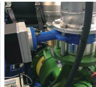
Servo control device to close delivery Valve
