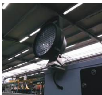
Light on pump side
