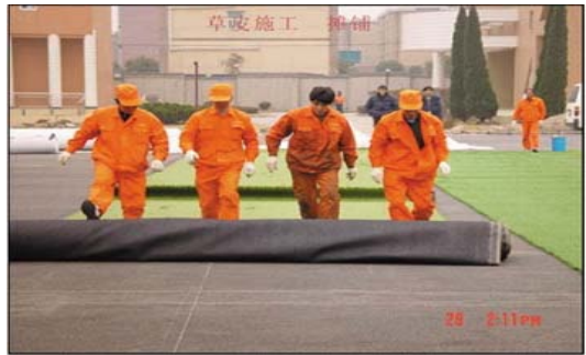
2: Unfolding the grass to both sides
