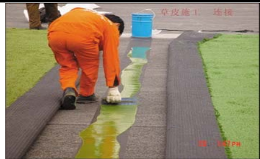
4: Jointing the tape and coating glue on the tape
