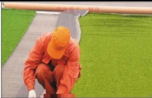
3: Cutting and trimming the grass edge
