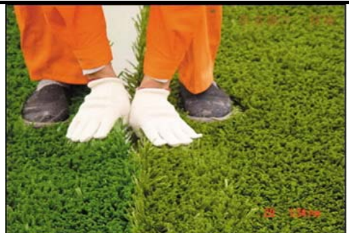
5: Offer the grass edge together and flattening the grass
