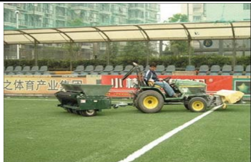
7: Filling rubber granule
